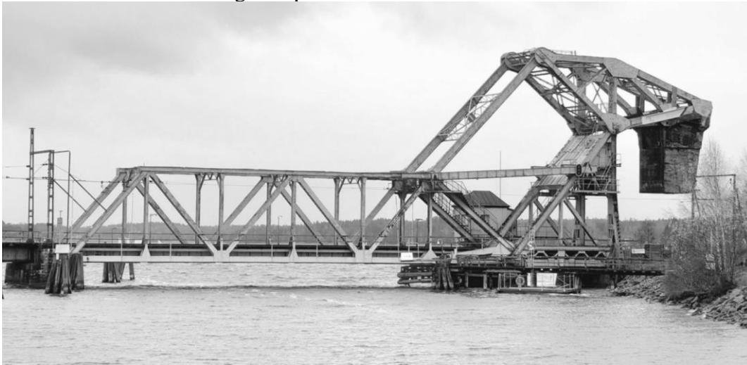
Figure 1. View of the case study of the steel-bascule-railway bridge
