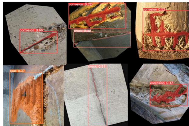
Figure 5: Incorrect detections and classifications of damages
